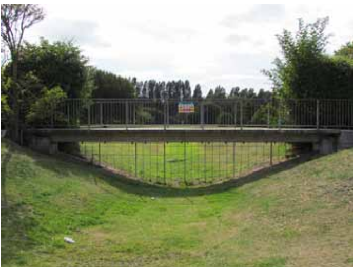
Drainage channels in Hall Place Gardens are designed to take overflow water if the river floods © Rory Walsh
