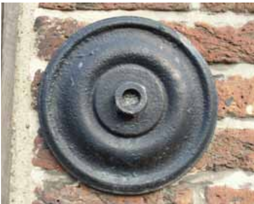
Look for the iron bolts holding on the façade © Rory Walsh
